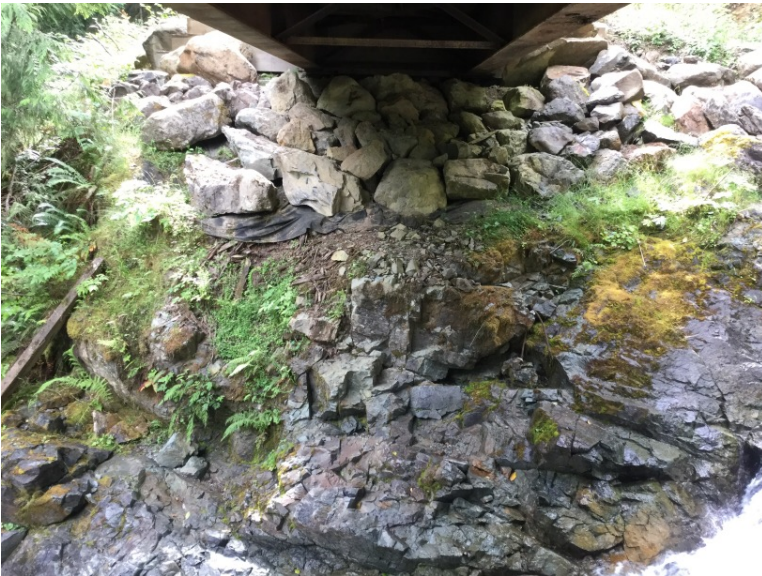
Right Bank Abutment when facing downstream
