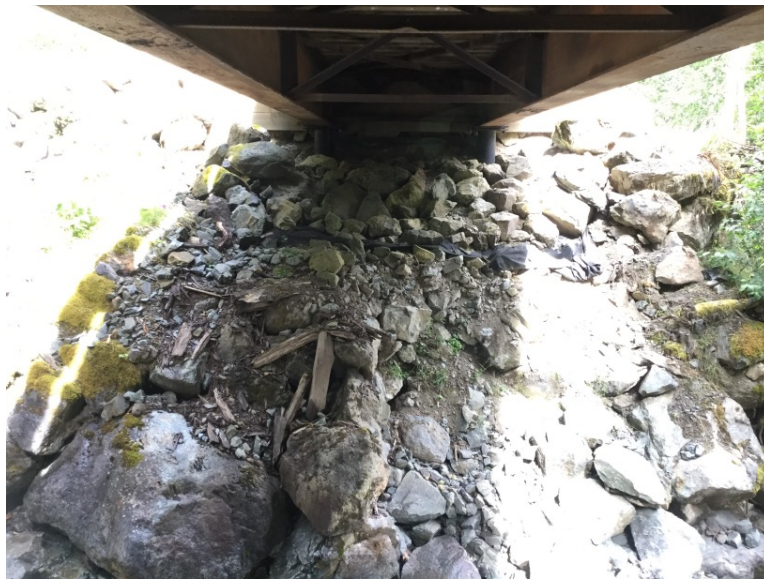
Left Bank Abutment when facing downstream
